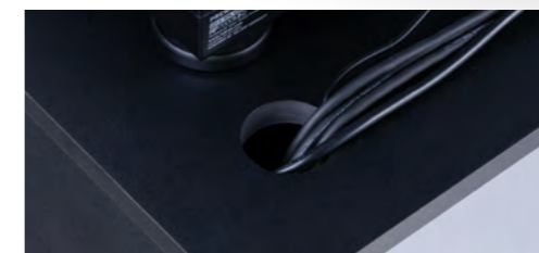
Various ducts for cable routing
